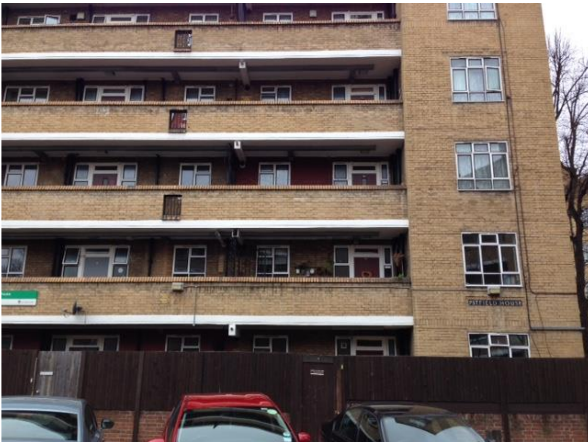
Image 3: view looking at the front façade of Pitfield House
